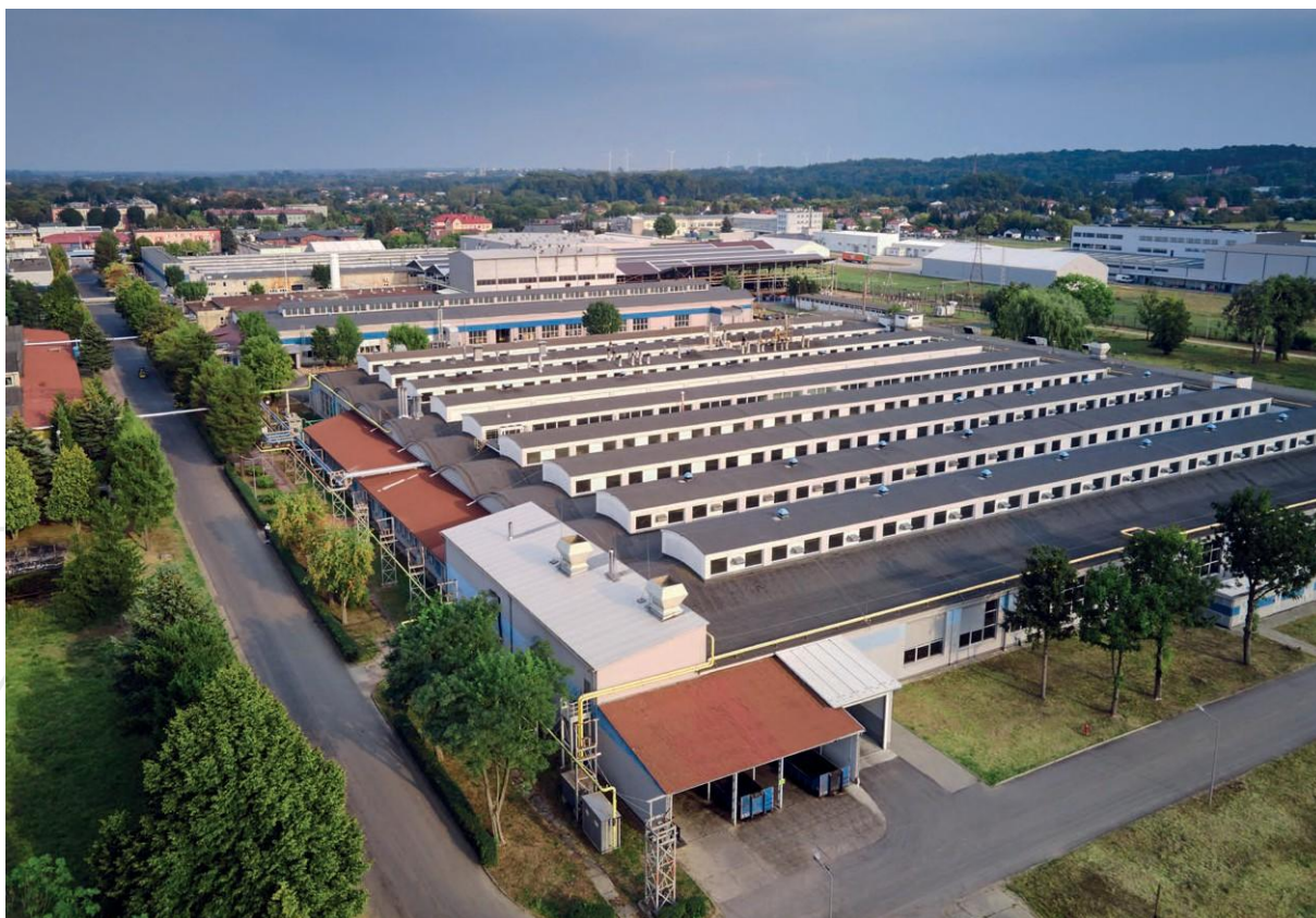
Figure 1. Production plant in Łańcut
