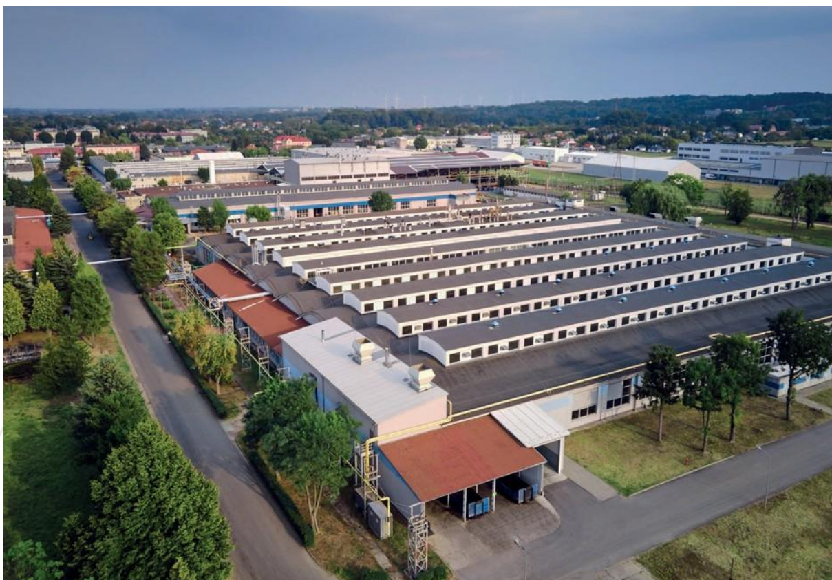
Figure 1. Production plant in Łańcut
